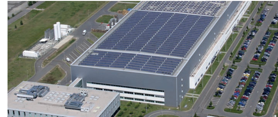
The highly efficient production lines at this site enable a cost-efficient production. The production costs in Frankfurt (Oder) are yet below the generally applicable solar module minimum price of 57 Cent per watt for imports from China.
