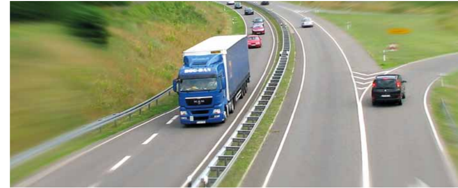
The large North/South connection on Oder-Lausitz-Road, just west of the River Oder, had been in construction for several years. The full Oder-Lausitz-Road route runs from the A11/A20 autobahn in the area south of Prenzlau via the cities of Schwedt, Bad Freienwalde, Frankfurt (Oder), Eisenhüttenstadt and Cottbus and constitutes the largest link road to the A13 autobahn.
